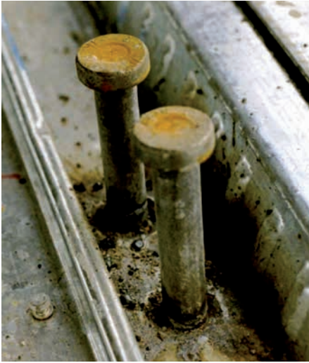
Figure 5: Shear studs welded on profiled deck
