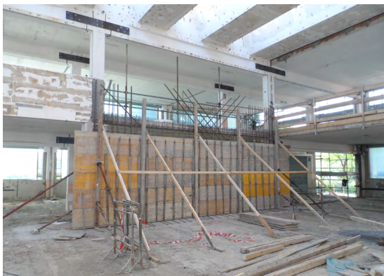
e) Shear wall addition
