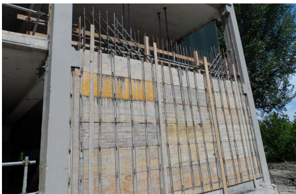
a) Corner walls
