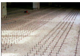
c) Slab strengthening with HCC-K shear connectors
