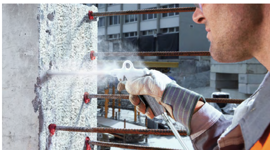
a) Air blow-out of dust from boreholes
