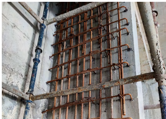
f) Structural wall strengthening
