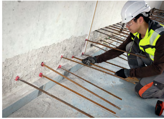
b) Slab-to-wall connection
