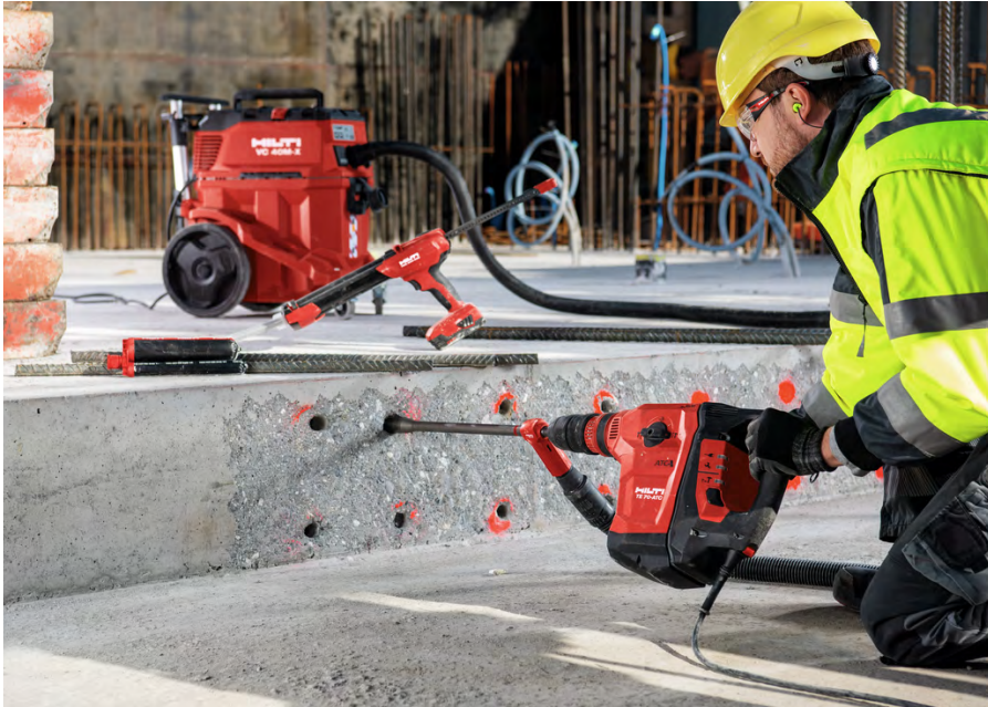
Fig. 9.16: Hilti SafeSet™ system – dust-free drilling of holes with hollow drill bits (HDB)
